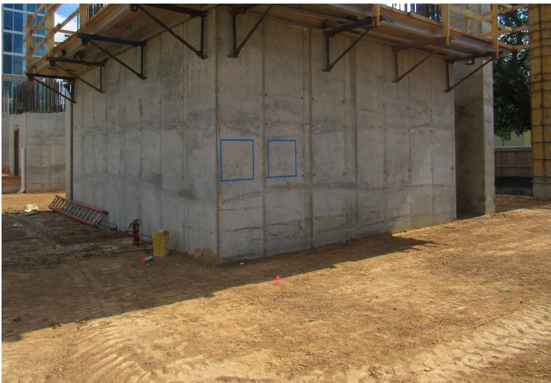
Fig. 6.20 Lab C shear wall with two sample areas taped off for measurement
