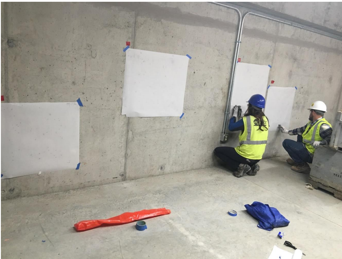
Fig. 6.10 Parking garage and office complex walls measured for SVR by MTSU student researchers
