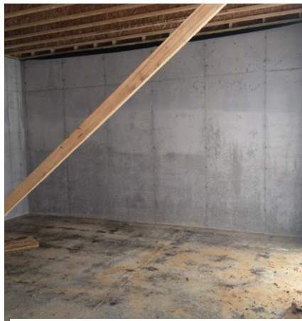
Small residence inside wall
